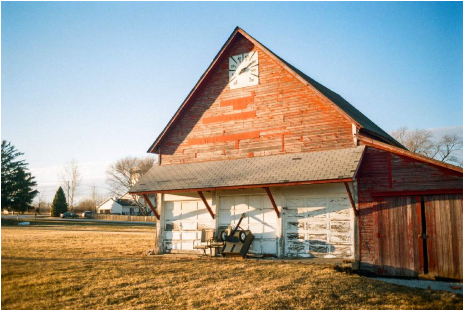
Barn Outside the Community Garden
